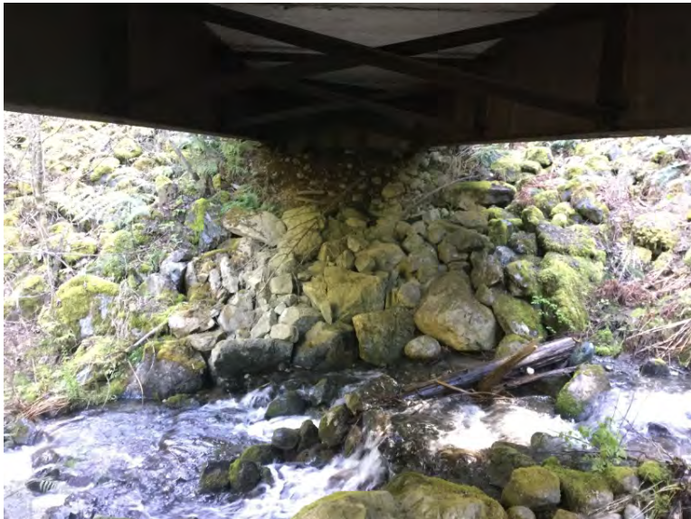
Right Bank Abutment when facing downstream
