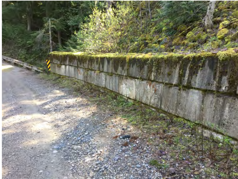
Fill retainment at upstream left approach, appears to be 3 blocks high
