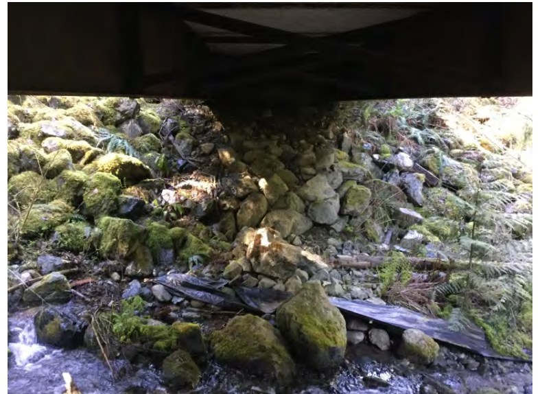
Left Bank Abutment when facing downstream
